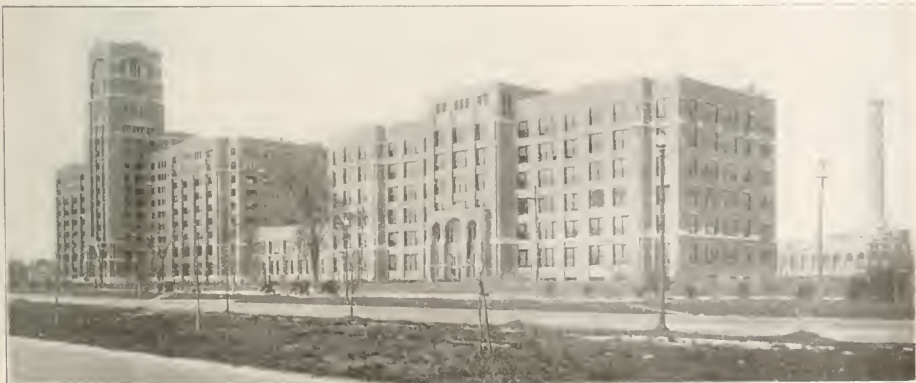
General view from Roosevelt Boulevard. The buttress construction of the Gothic is here appropriately adapted to modern industrial use.
